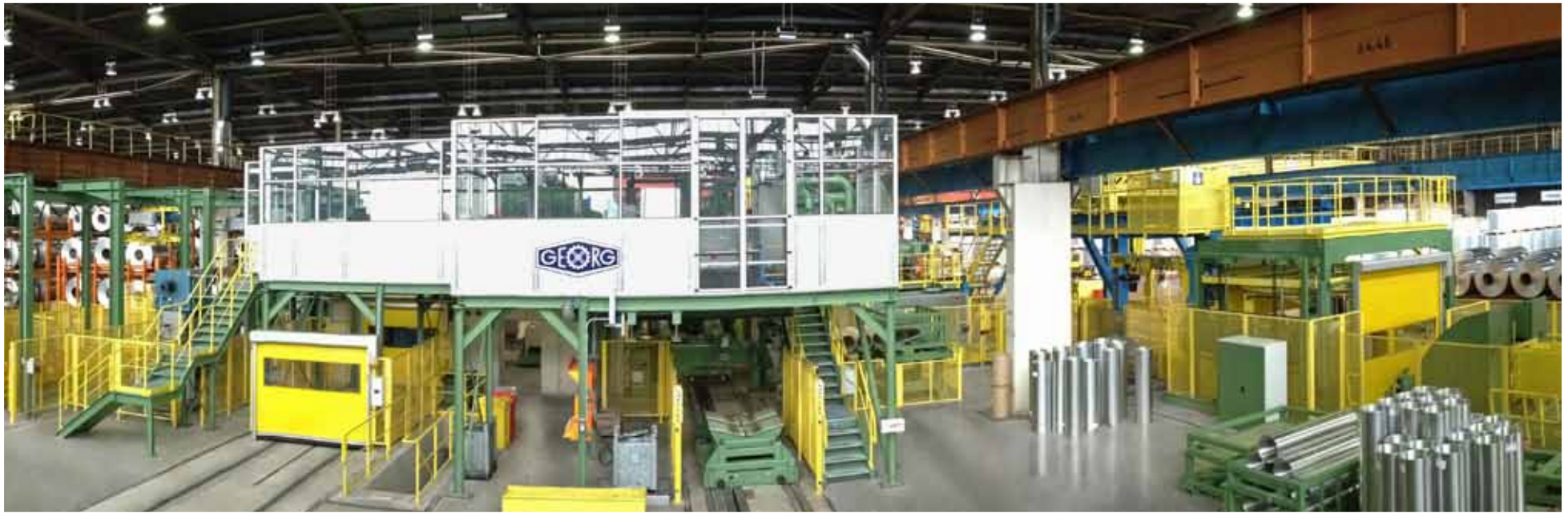
Edge-trimming line for aluminium with production speeds >1,800 m/min.
